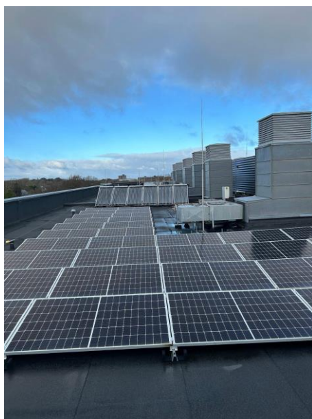
Figure 11. Alice Perry building's renewable installations (PVs and PVTs on the left and AHX on the right)
