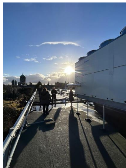
Figure 13. NUIG's Mathematics building heat pump installation (buffer tank and flow pipes on the left and AHX on the right with PVs in the background)
