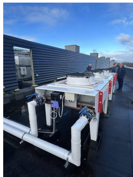
Figure 11. Alice Perry building's renewable installations (PVs and PVTs on the left and AHX on the right)
