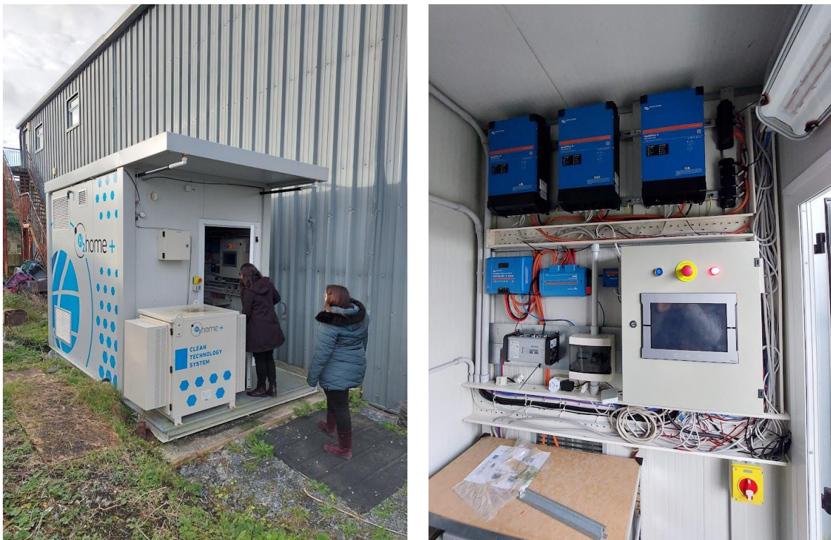
Figure 16. Innovative CTS-H2 system at the recycling center showing the fuel cell on the left and inverters and control unit on the right
