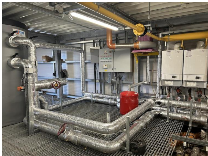
Figure 13. NUIG's Mathematics building heat pump installation (buffer tank and flow pipes on the left and AHX on the right with PVs in the background)
